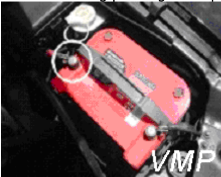
Wire orange wire to + battery side
